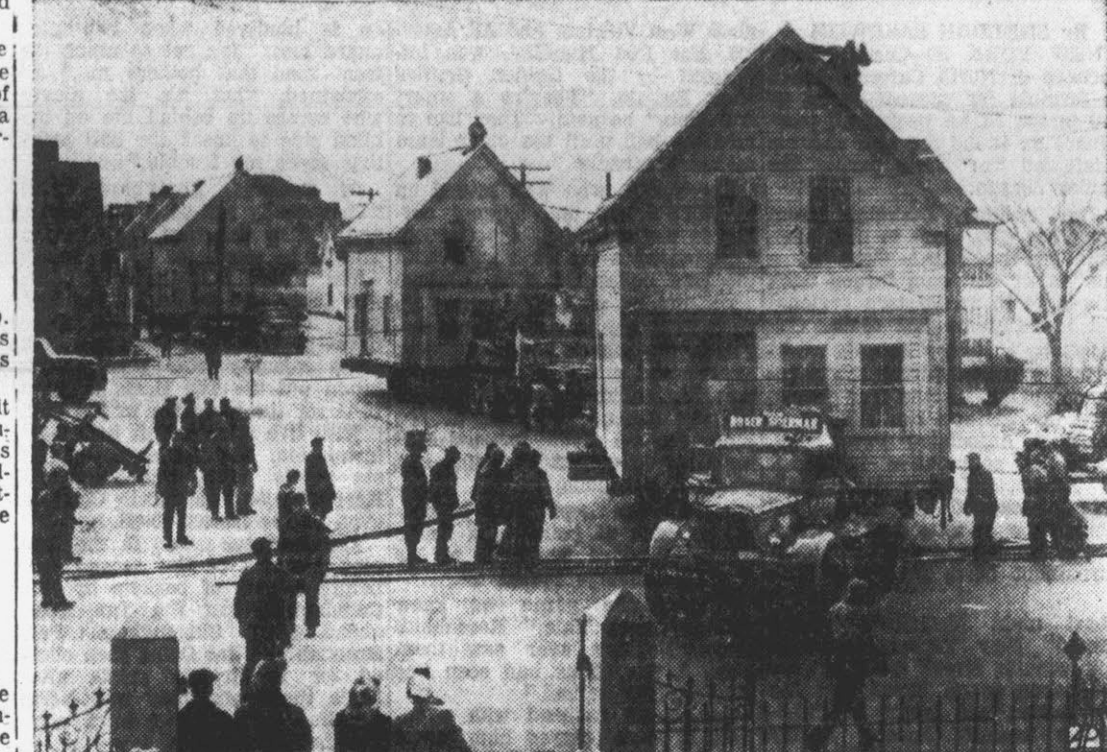
HOUSES ON THE MOVE—Four frame houses, on flat bed trailer trucks, form an unusual procession as they move slowly through a Lynn, Mass., street to their new location.
