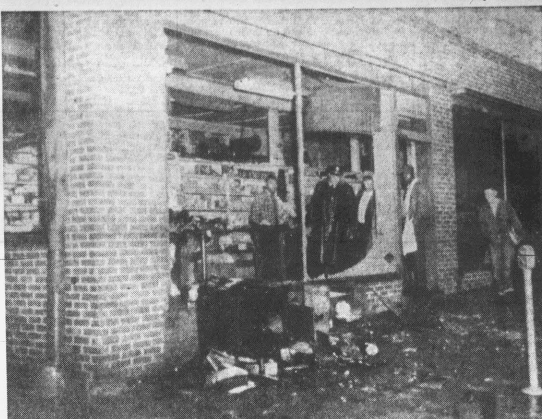
FIRE—An early morning fire damaged Bunch Shoe Shop on Cotanche St. today. The fire, believed started from an oil stove, was confined to the front of the building.
