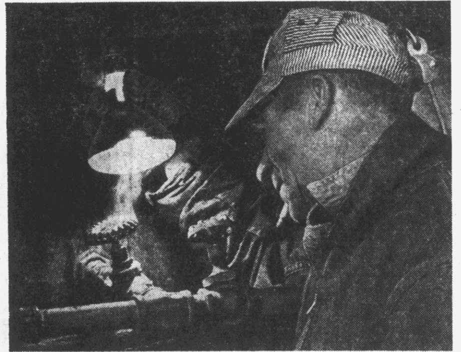
Heat lamp is a must during cold winters to keep water valves workable. Brockman checks valves on his storage tank.
