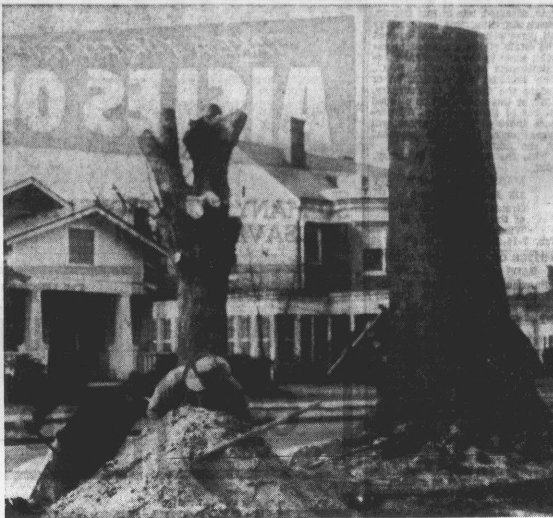
DOWN THEY GO—Workmen are shown above removing one of the old shade trees on Evans Street. In the background is a tree that had been topped by workers yesterday morning. A large number of trees on the local street have been topped and will be uprooted in the near future as the city plans to widen Evans Street in the future. (Reflector Staff Photo).
