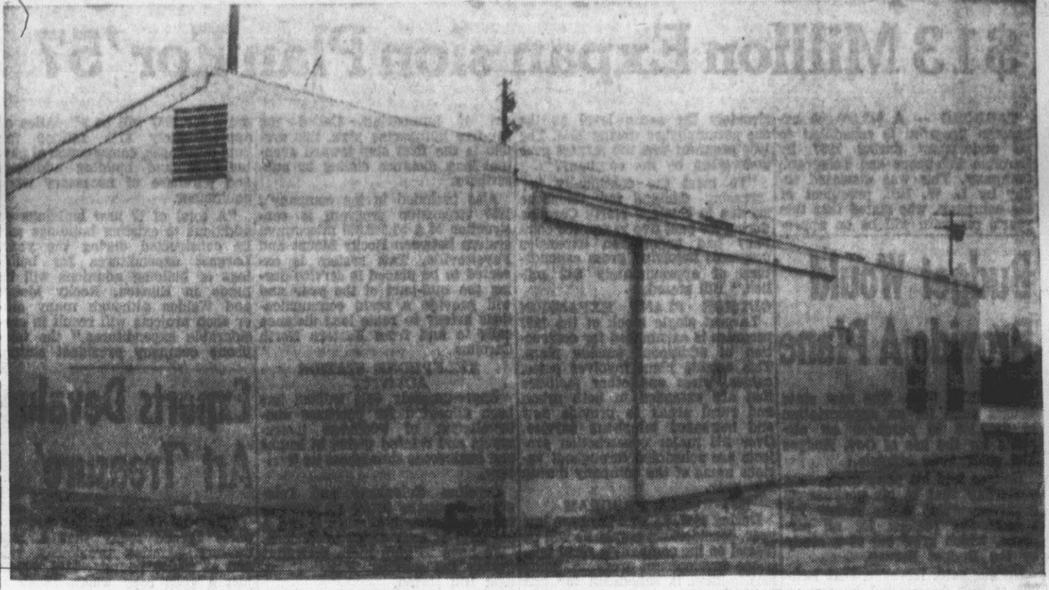
NEW RECREATION SHOP—This metal building has recently been constructed at Guy Smith Park for use as a shop and storage building for the Recreation Department. Some $5,000 was approved in a recent bond issue for construction of the building. (Reflector Staff Photo).
