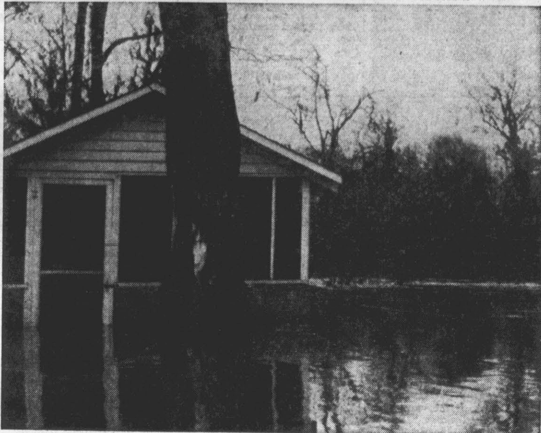
Tar River has invited itself into Frank Dall's picnic house at the foot of Jarvis Street. Ordinarily, the little house stands high and dry on the south bank of the river but when the water rose to 13.79 feet yesterday water was about two feet deep inside. The river is expected to crest at about 18 feet tomorrow night—about five feet above flood stage. (Reflector Staff Photo).
