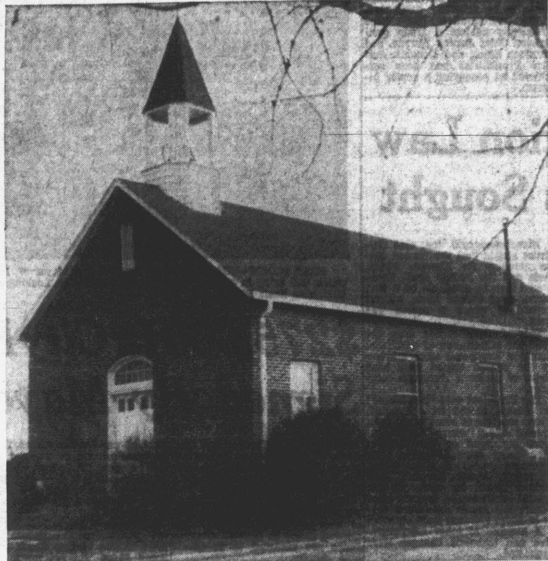
QUITE PROUD—The little Methodist Church of Stokes sits quite proudly on Route No. 903. It isn't everyday that a little country church gets over $40,000 worth of publicity, new pews, new ceiling, a stove, refinished floors, a new communion table, and has its chancel divided.
