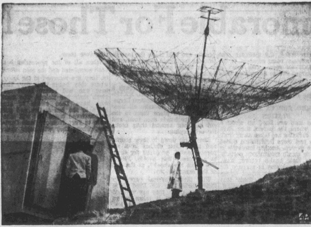
SIGNAL INFORMANT—Huge parabolic antenna is readied at Palo Alto, Calif., for shipment to Alaska to gather information about reflection of VHF and UHF radio signals.
