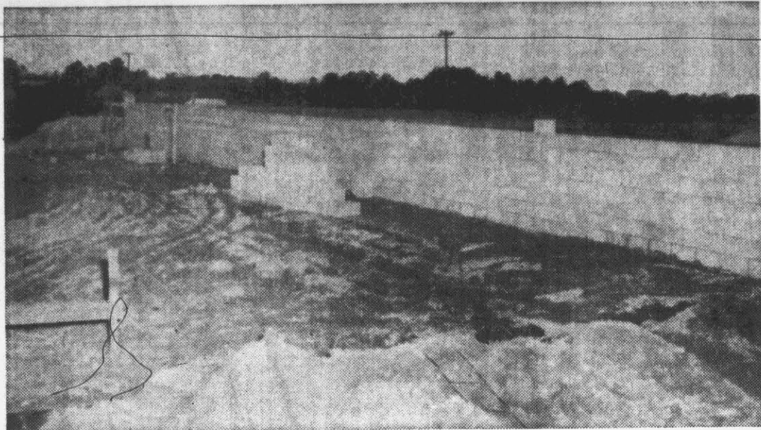
PROCESSING PLANT CONSTRUCTION —Construction of the new Austin Farms, Inc. plant formerly of Wendell, is showing much progress in Robersonville despite inclement weather during the first part of January. The foundation, contracted by E. L. Rackley of Raleigh, is near completion to pave the way for the Strand steel to be erected, weather permitting, in the next 30 days. Pictured above are two scenes of the building that were taken earlier this week in the Martin County community. The plant is scheduled to be completed sometime during the month of May. Broiler chickens will be processed for commercial use and will be contracted and sold to points throughout this and neighboring states. (Reflector Staff Photo).
