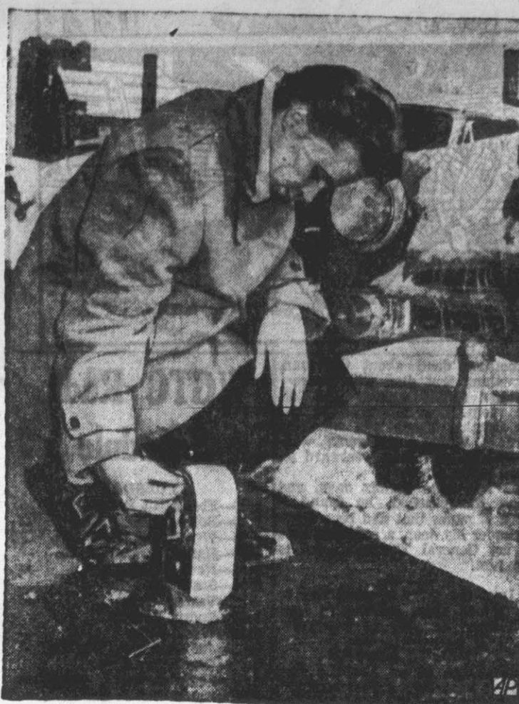
Phyllis Hutchins puts a coin in a Michigan City, Ind., parking meter Jan. 12, though she isn't sure it will be there when she returns. It was found meter is sinking into a coal chute beneath the sidewalk. (AP Wirephoto).
