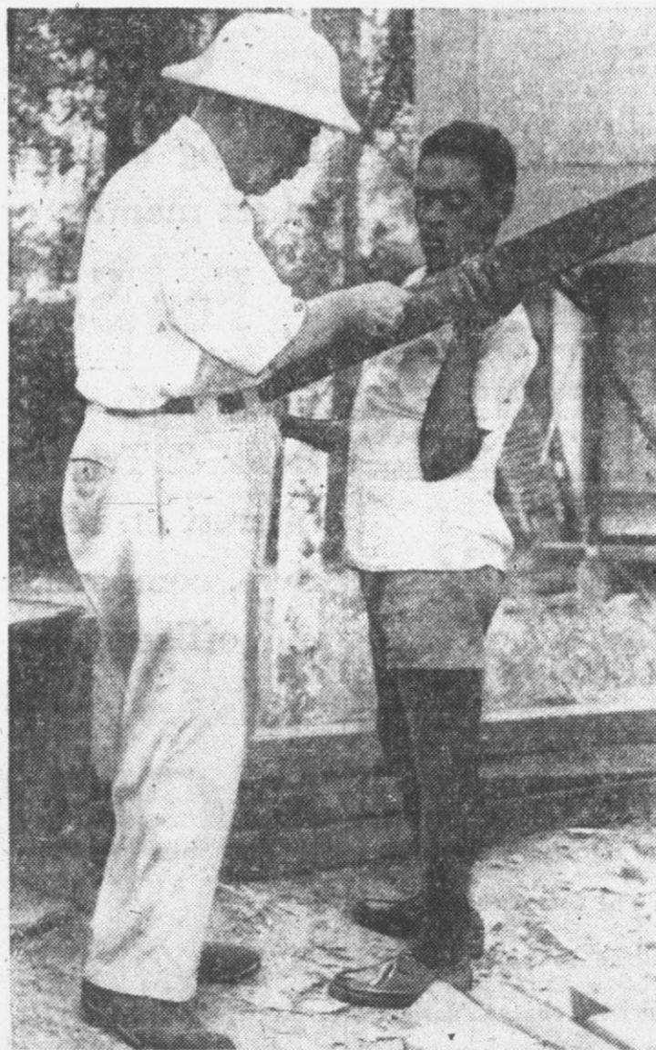
A vigorous man, despite his years, he helps with construction of new building for his colony.
