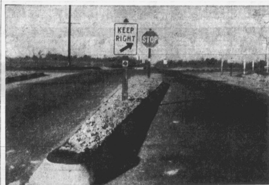
IMPROVE INTERSECTION—State Highway Department work crews have recently improved the intersection of Evans St. Ext. and the U. S. 264 bypass. Traffic islands have been built and stop signs placed in the center of the road on Evans St. Ext. The intersection has been the scene of several serious traffic accidents. (Reflector Staff Photo).
