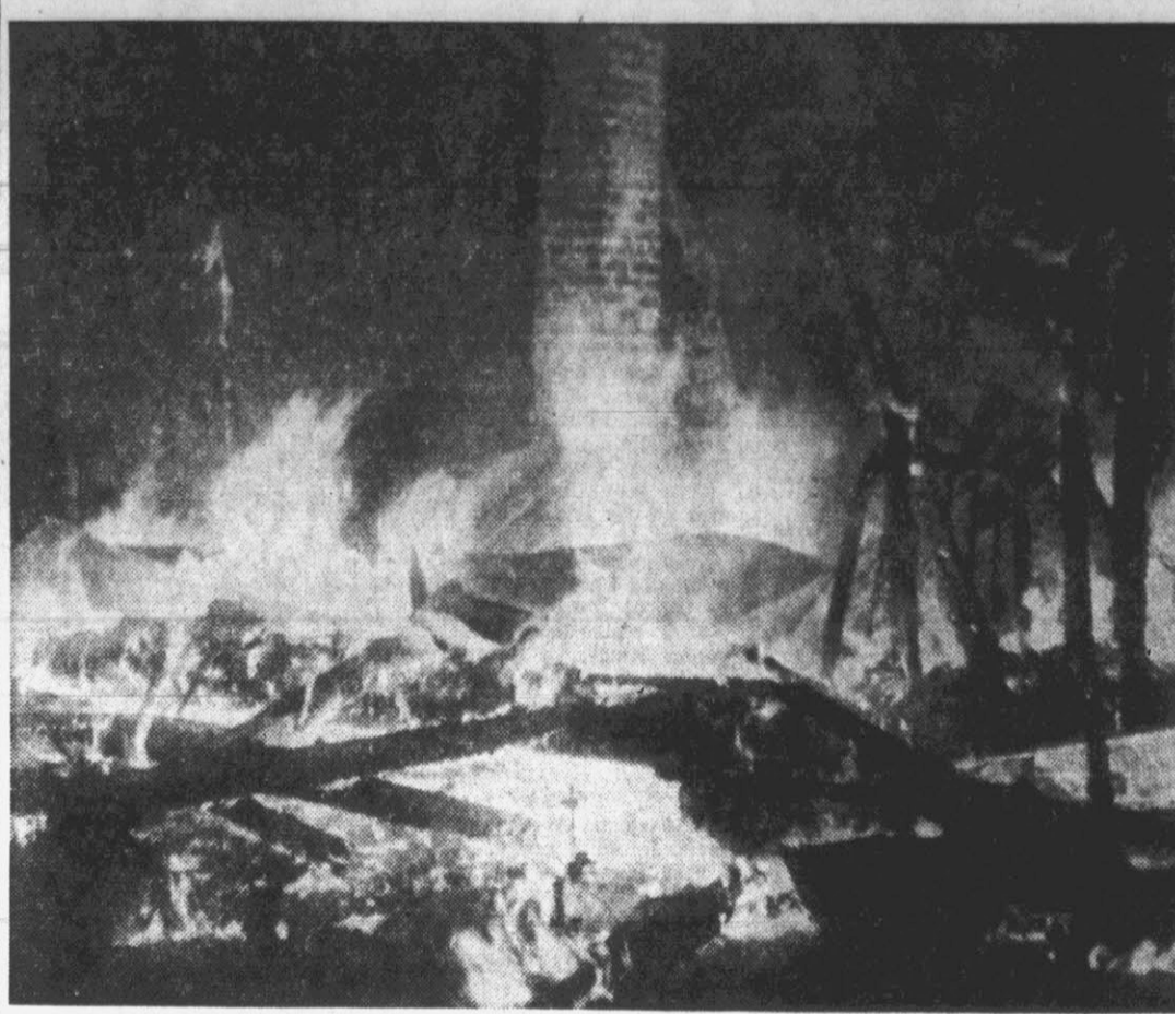
FIRE—Flames destroyed this house shortly after 5 o'clock yesterday afternoon. The dwelling was owned and occupied by John Henry Davis, 73-year-old Negro. No one was home when the fire broke out. (Reflector Photo by Alvin Taylor).
