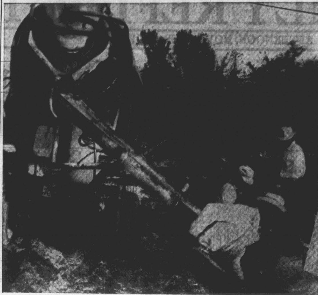
STREET WORK BEGINS —Workmen are shown above as they pour concrete for curbing on Elm St. The work on that street began last week and it is the first of the street paving and curb and guttering program to be carried out this year with Powell Bill funds. Elm St. is to be paved from Third St. to the city limits. In addition one block of Oak and a block of Third to Oak will be paved and curb and gutter installed. Curb and gutter is to be placed on W. Fifth St. from Forest Circle to Cedar St. And paving and curb and gutter is to be placed on Bonner's Lane and Atlantic Ave. (Reflector Staff Photo).
