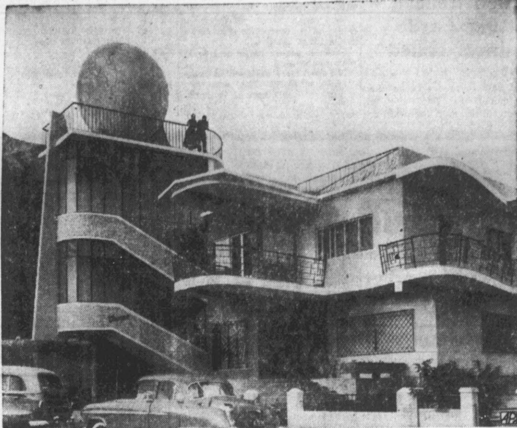
SERVING DOUBLE PURPOSE —A hollow replica of the planet Earth atop this Caracas, Venezuela, home provides a geography lesson besides serving as the family's water tank.
