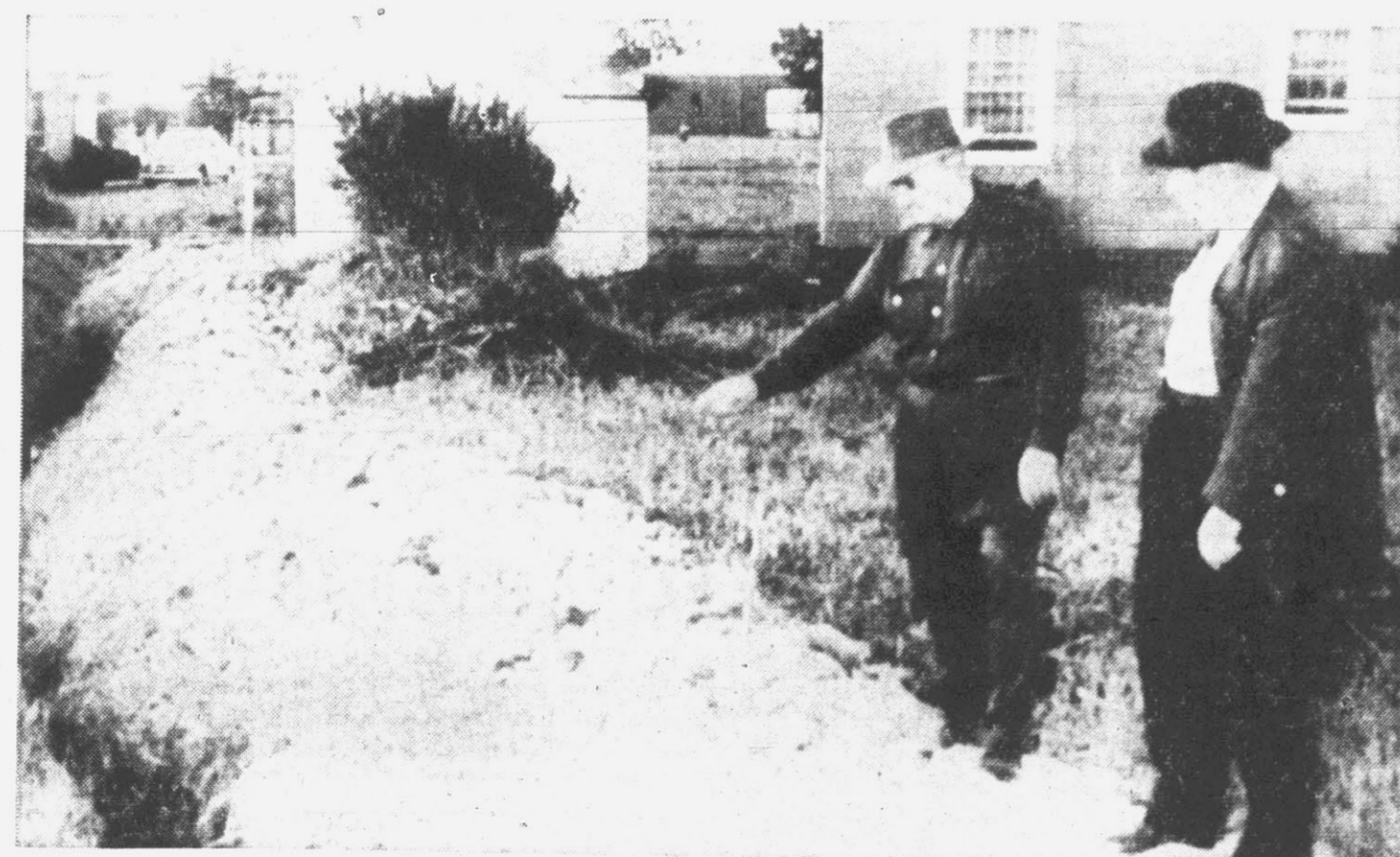
DITCH TO BE ELIMINATED —Public Works Superintendent Beatty and City Manager Bloxam look over a ditch which will be eliminated under the storm drainage portion of the proposed bond issue. Some $187,000 would be spent on storm drainage if approved.
