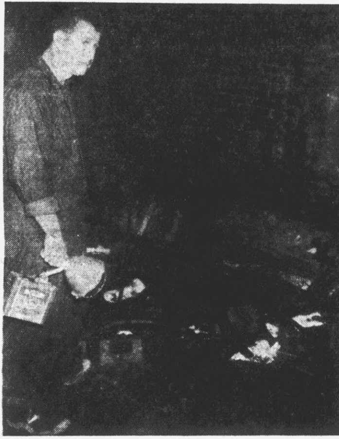
POINTS TO BODY—Fireman Amos Harrell shines a light on one of the two bodies found in the wreckage of the Dixie Warehouse. (Reflector Staff Photo).
