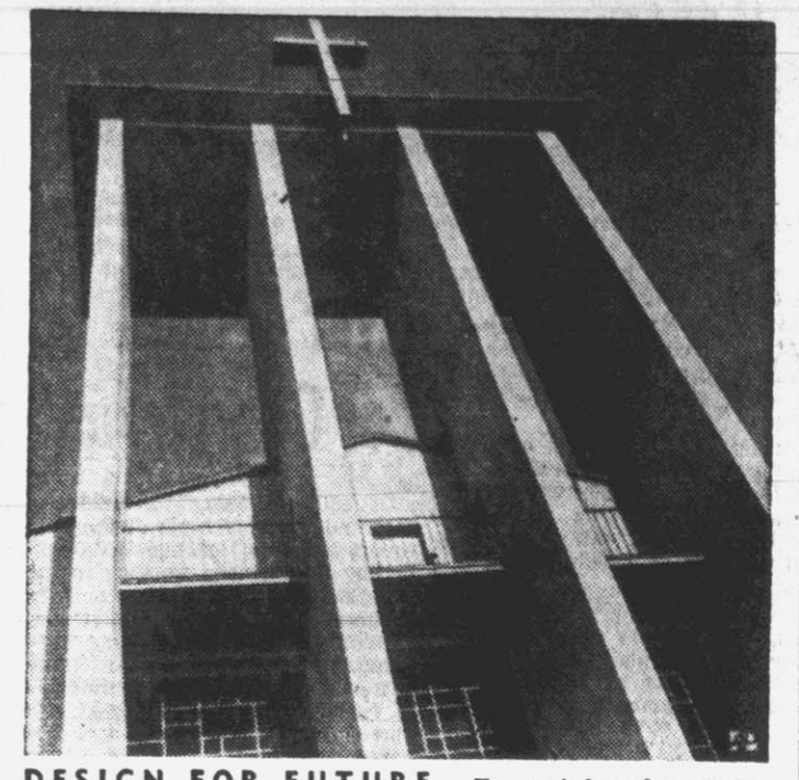
DESIGN FOR FUTURE — Four reinforced concrete columns, between which bells will be suspended, form the steeple for a new Catholic church in Frankfurt, West Germany.
