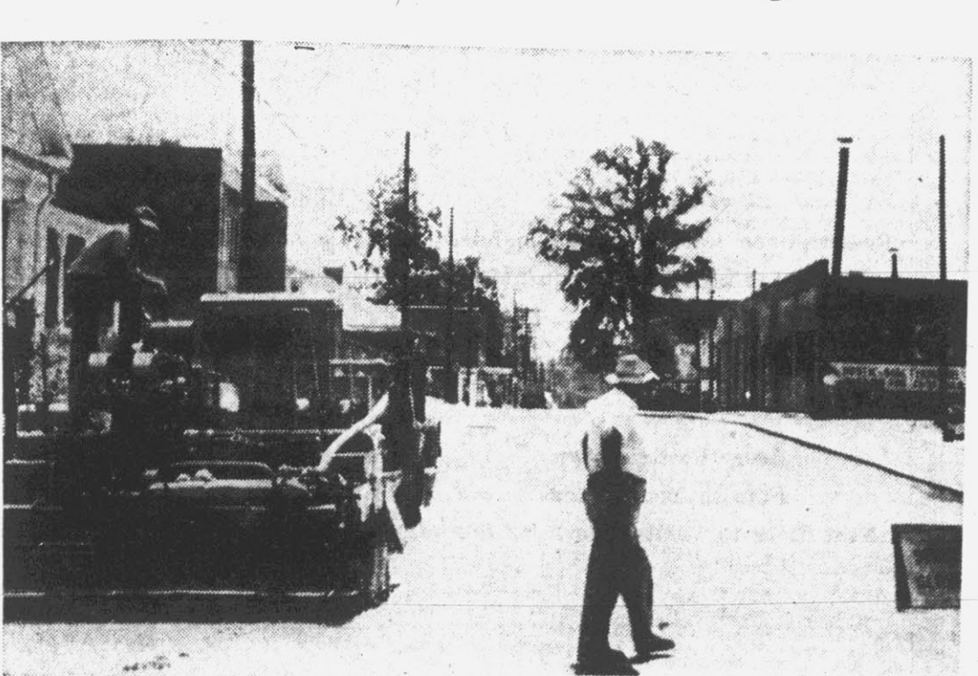
PAVE BLOCK - Workmen yesterday paved a block of Cotanche St. between Second and Third Sts. The block was recently widened after property owners deeded land needed for the job. The city also installed underground conduits on the block to be used later when other conduits are placed under downtown streets. (Reflector Staff Photo).
