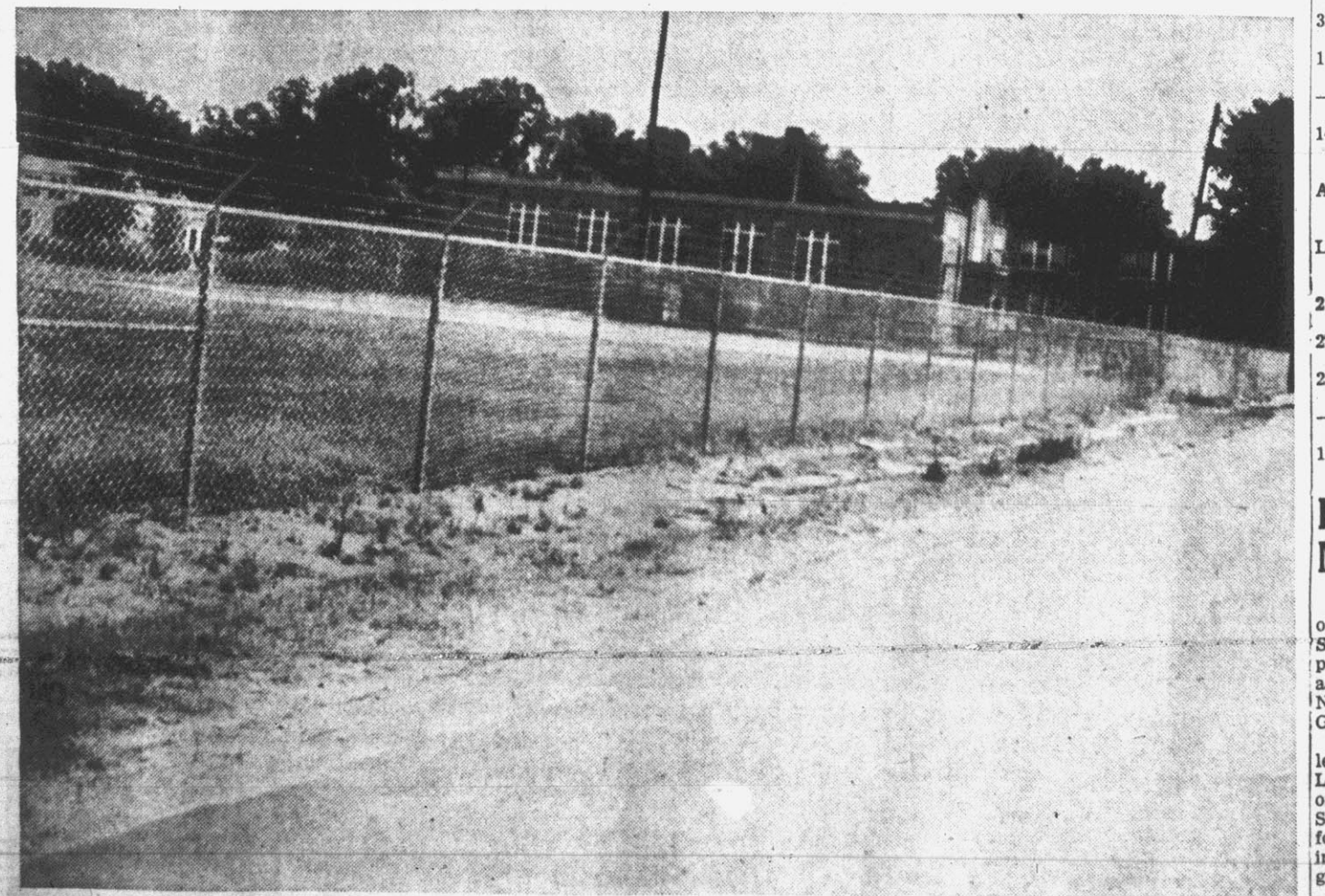
A new cyclone wire fence has been erected around the Ayden High School athletic field to replace a six-year-old wooden fence which was destroyed by hurricanes last year. The new fence cost $2,440, including installation, under a contract price. The wooden fence which formerly enclosed the athletic field cost $2,000 when it was put up in 1950. (Reflector Staff Photo.)
