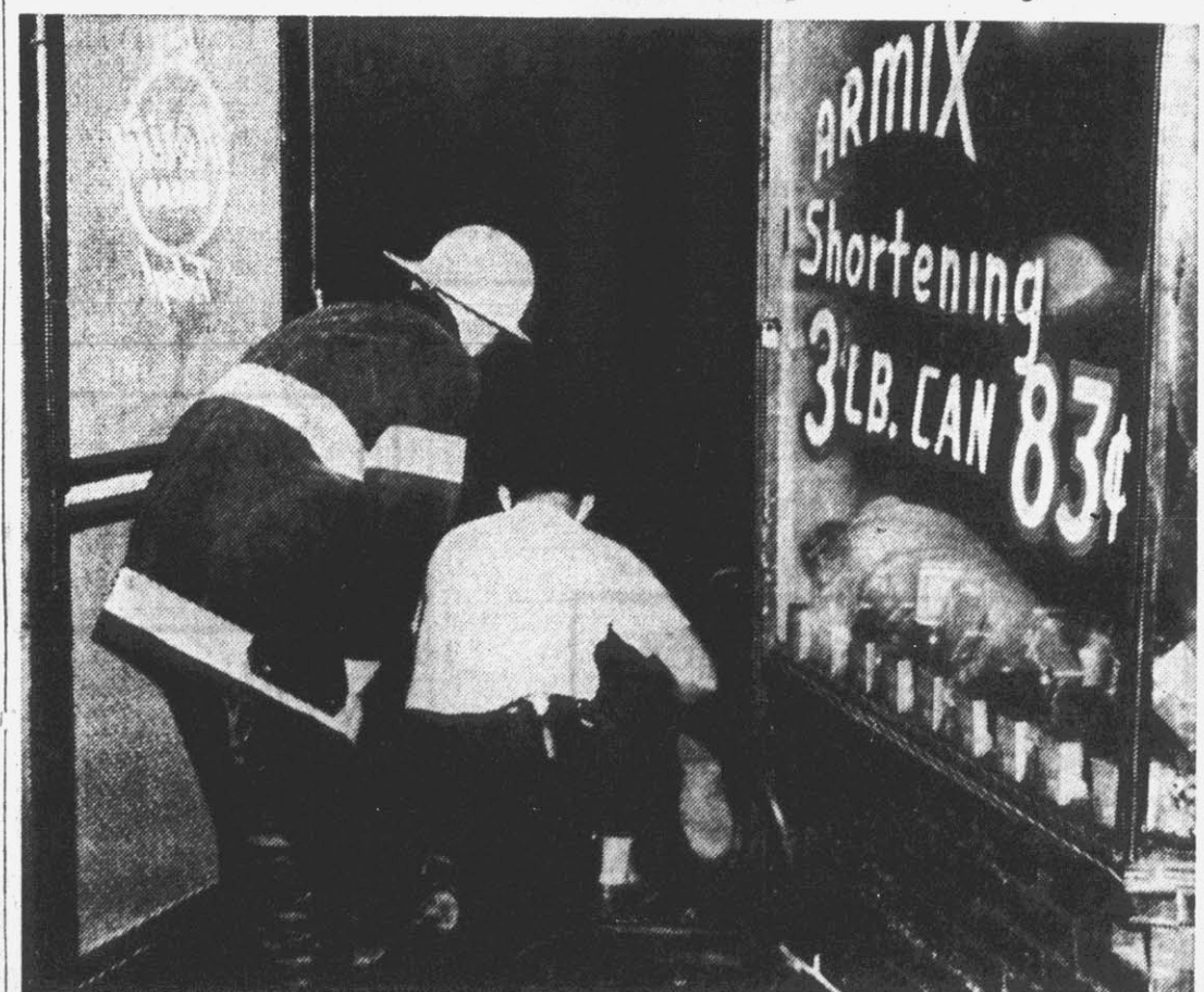
ENTER STORE—Firemen are shown above as they enter Honeycutt's Market to fight a blaze which broke out in the store early Sunday morning. The fire which apparently began in a freezer unit, was quickly extinguished. Fire damage was largely in and around the freezer unit. (Reflector Photo by Alvin Taylor)
