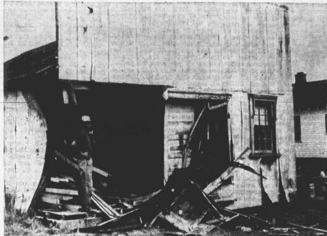
HOUSE DAMAGED—Robert Harrell of 700 Tyson St. stands in the gaping hole left in the front of his home when an automobile crashed into the front of the structure last night. Harrell and his wife were sleeping in the rear of the house and were unharmed by the crash. Damage to the house was estimated at $1,500.
