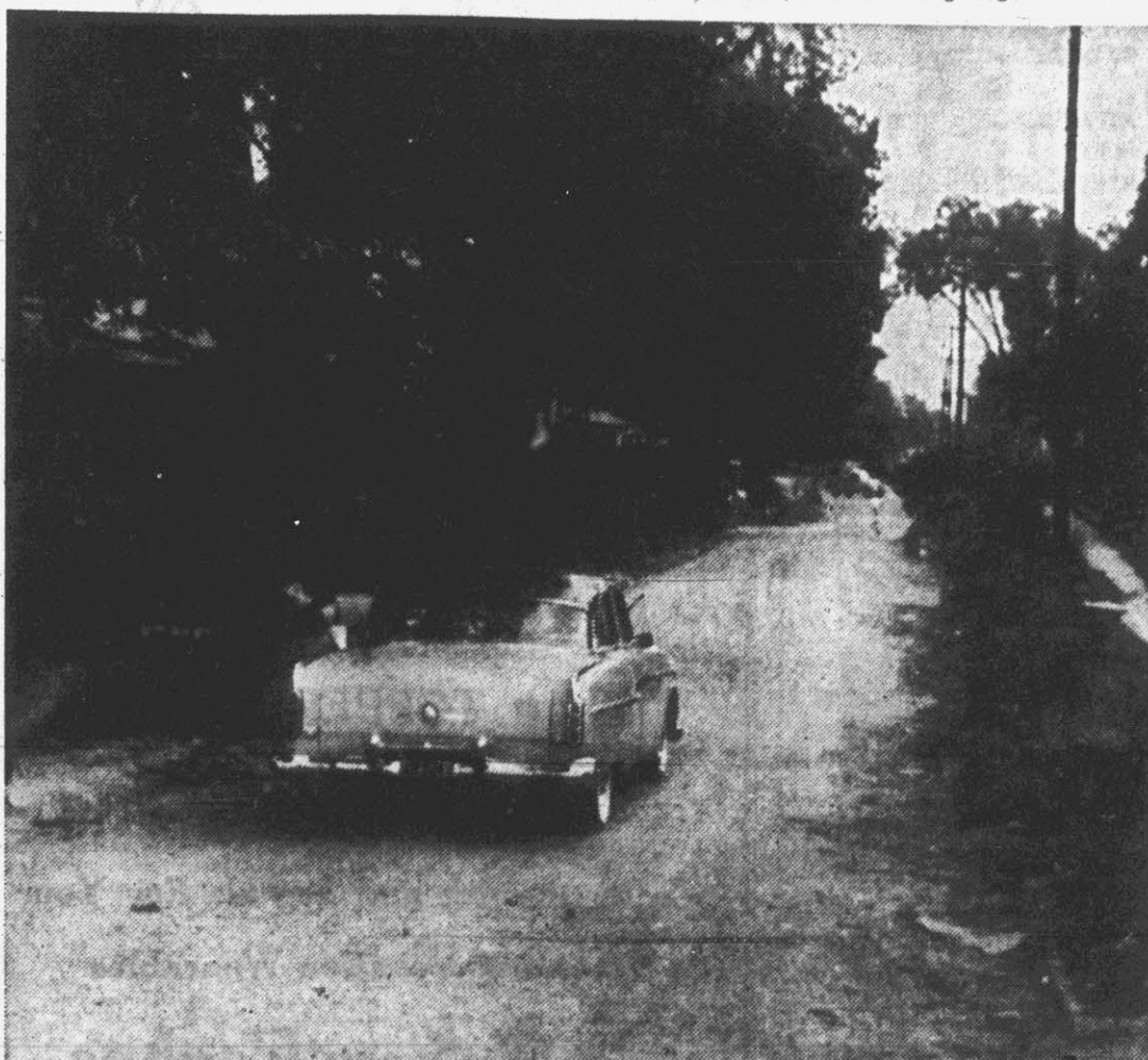
FIRST STREET—This portion of First St. which will be widened and curb, gutter and paving installed if approved by the voters in the bond issue election of July 10. The work also includes the construction of a fill for First St. (Reflector Staff Photo).
