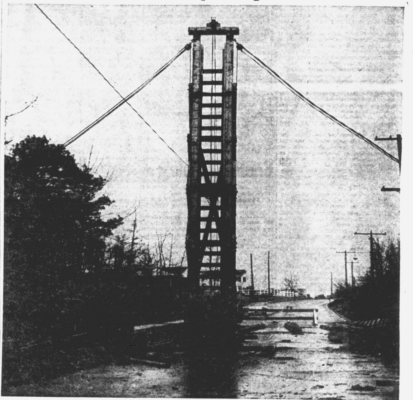
This towering pile driver creates a striking break in the skyline on 14th St. This device is being used for rebuilding the Greene Mill Run bridge on that street. Work is being done by Highway Department crews. (Reflector Staff Photo).
