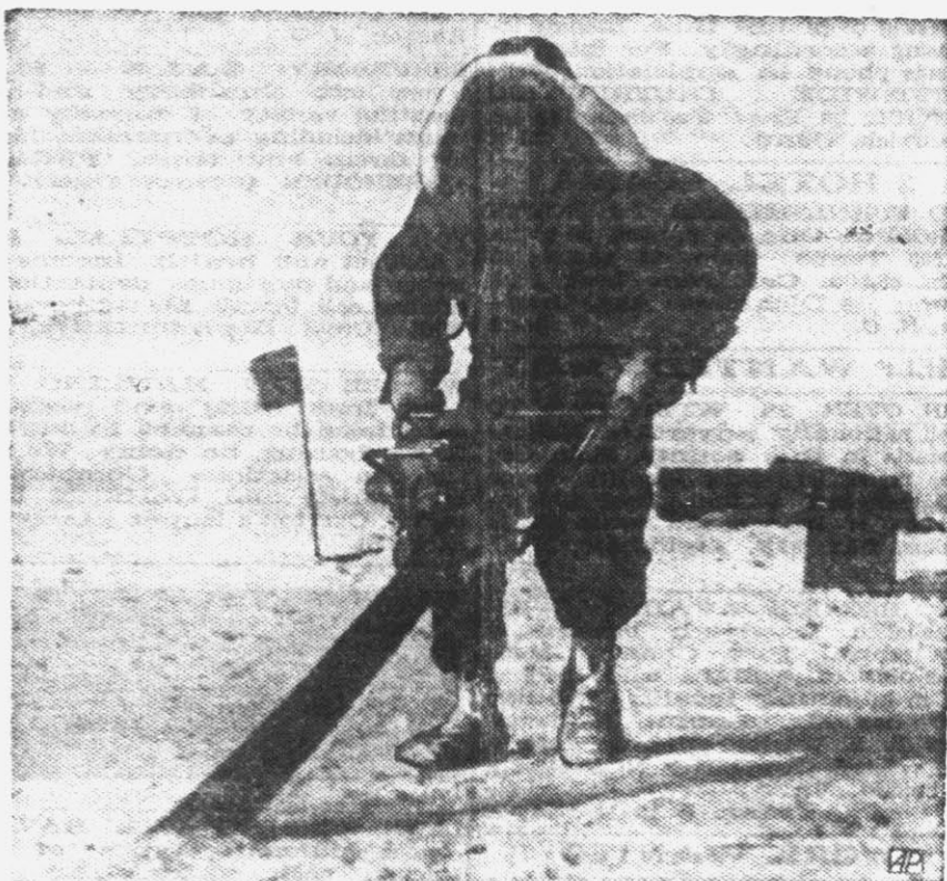
ANTARCTIC ICE CHECK—A Seabee with U.S. Navy's Antarctic expedition tests ice thickness on McMurdo Sound with seven-foot power saw for possible airfield location.
