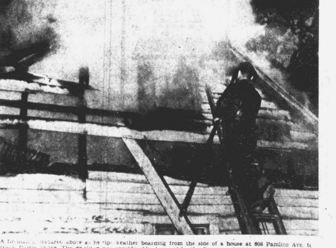
A fireman is pictured above as he rip weather boarding from the side of a house at 808 Pamlico Ave. to reach flames in the dwelling which was considerably damaged by the fire around midnight last night. (The Reflector Photo by Avim Taylor).
