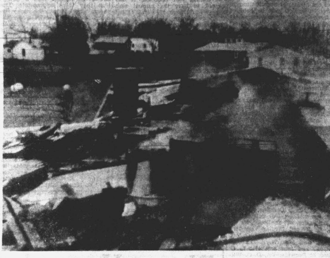
AS BLAZE DIED DOWN The collapsed roof of Ayden's new medical clinic smoulders early today after fire raged through the $60,000 building doing heavy damage. Firemen from Greenville and Ayden fought the blaze almost three hours. (Reflector Photos by Bob Hillrup.)
