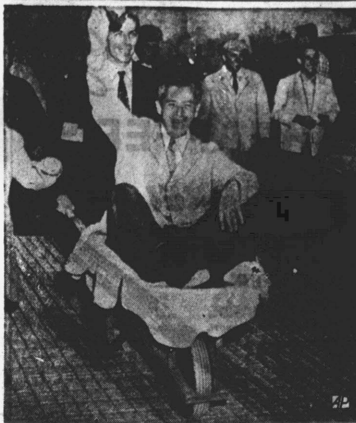
GOVERNOR TAKES A TRIP—Gov. LeRoy Collins of Florida grins broadly and waves as he rides in a wheelchair across a new bridge just completed across the Inland Waterway at Pompano, Fla. It's something new in dedication ceremonies although the governor cut the conventional ribbon before going for this somewhat unconventional ride as the first passenger across the bridge. (AP Wirephoto).
