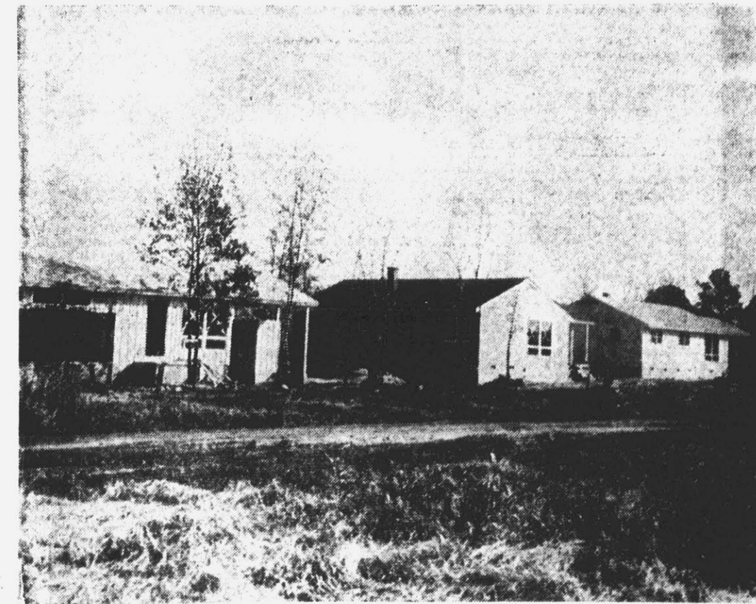
The third housing project since 1951 in Grifton is presently underway in that town. Six houses of the proposed 42-unit project are now under construction involving an estimated $65,000. The houses are seven-room dwellings and are being built of asbestos shingle and brick.
