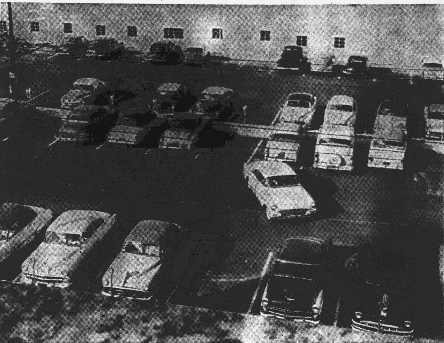
Pictured above is the first of the city's three off-street parking lots. It was constructed over the old swimming pool on Fifth Street. The unused pool was filled in and spaces were marked off for parking. The lot is unmetered and it is usually filled during the day. (Reflector Photos by Alvin Taylor).
