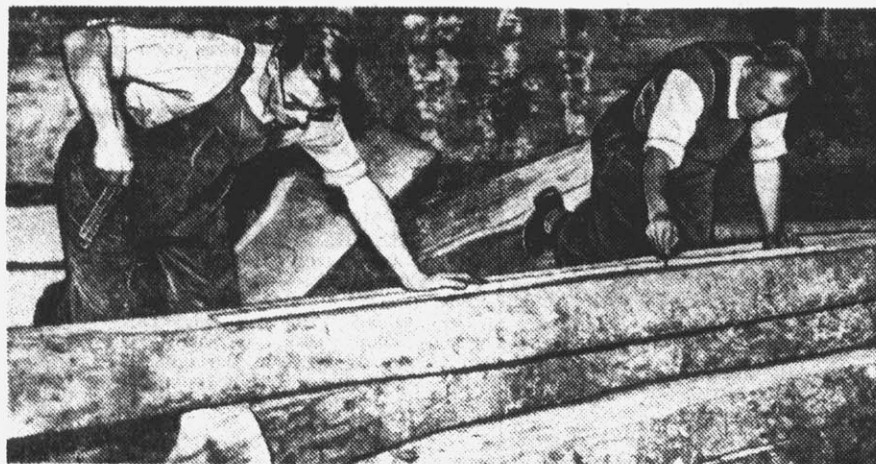
Carpenters at Brixham shipyard measure rough-hewn planks of English oak for "conversion," or shaping, for the new Mayflower.
