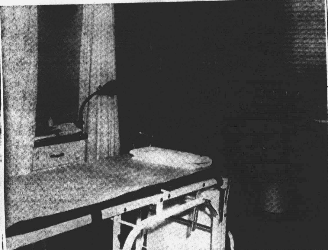
There are four examination rooms like this one in the new health building. This means that more patients can be treated with greater facility during the clinics. Each examination room is fully equipped with examination table, dressing cubicle, cabinets, sink and counter space.
