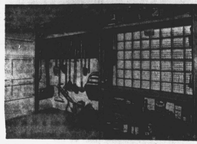
AFTER—A minor alteration, replacing the window with a panel of glass blocks, and rearranging available space, storage needs were filled and the efficiency of the garage was increased. The glass blocks spread light throughout.
