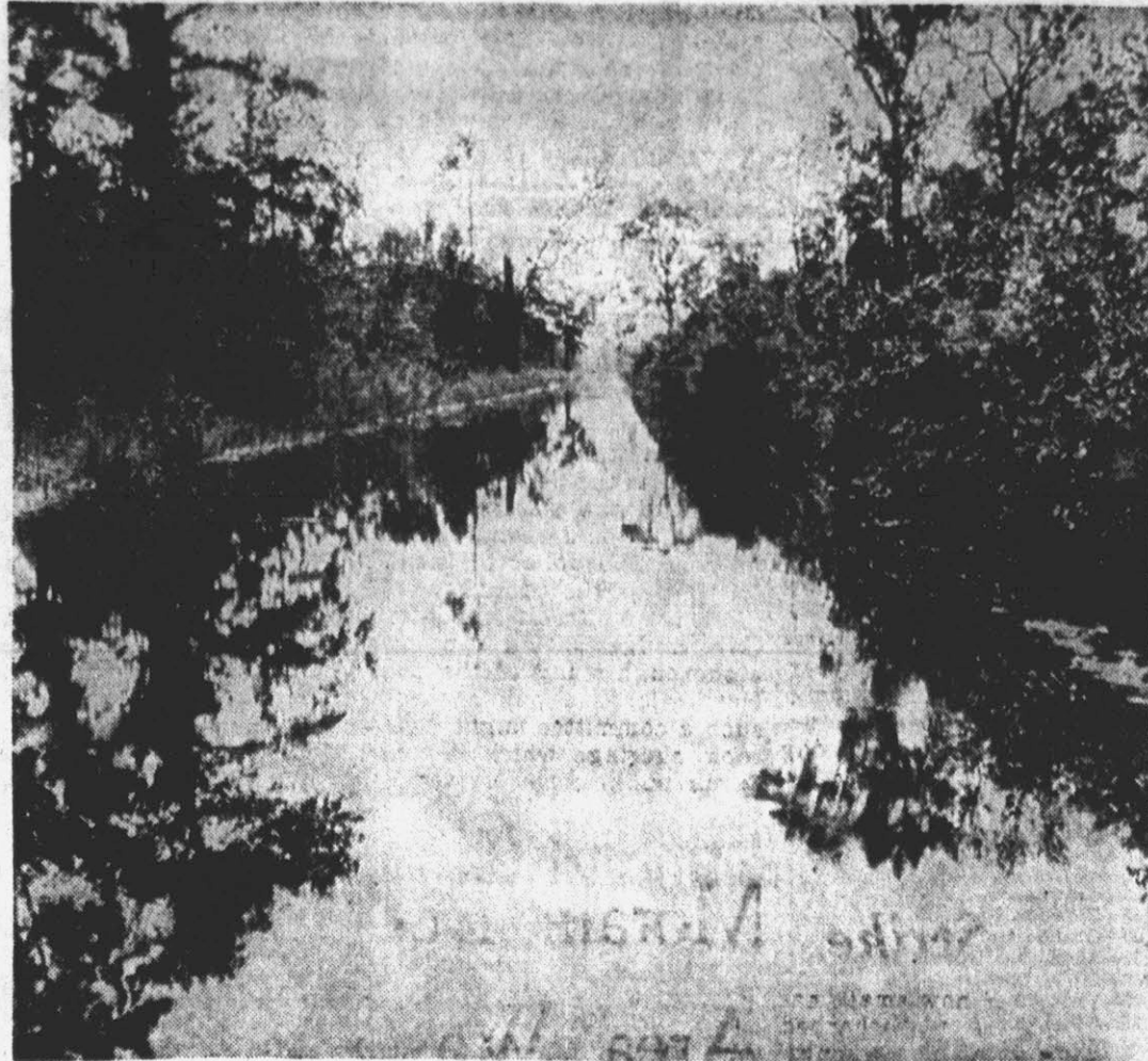
BLOCKED ROADWAY —This public road near Bethel is blocked often for stretches of more than a half mile simply because the Grindell Creek Canal is so choked with debris as to prevent the handling of water brought into it by drainage ditches dug by farmers. A project is planned to clear the canal and prevent future flooding such as this.
