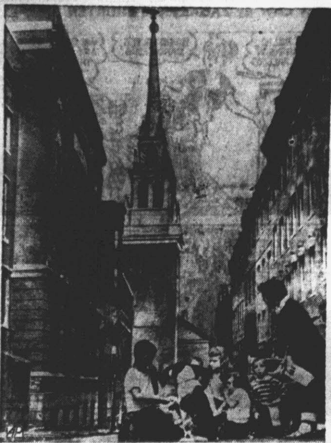
ONE YEAR LATER — Children play near Old North Church, Boston, shown with new steeple replacing one toppled by hurricane a year ago. New one is believed hurricane-proof.
