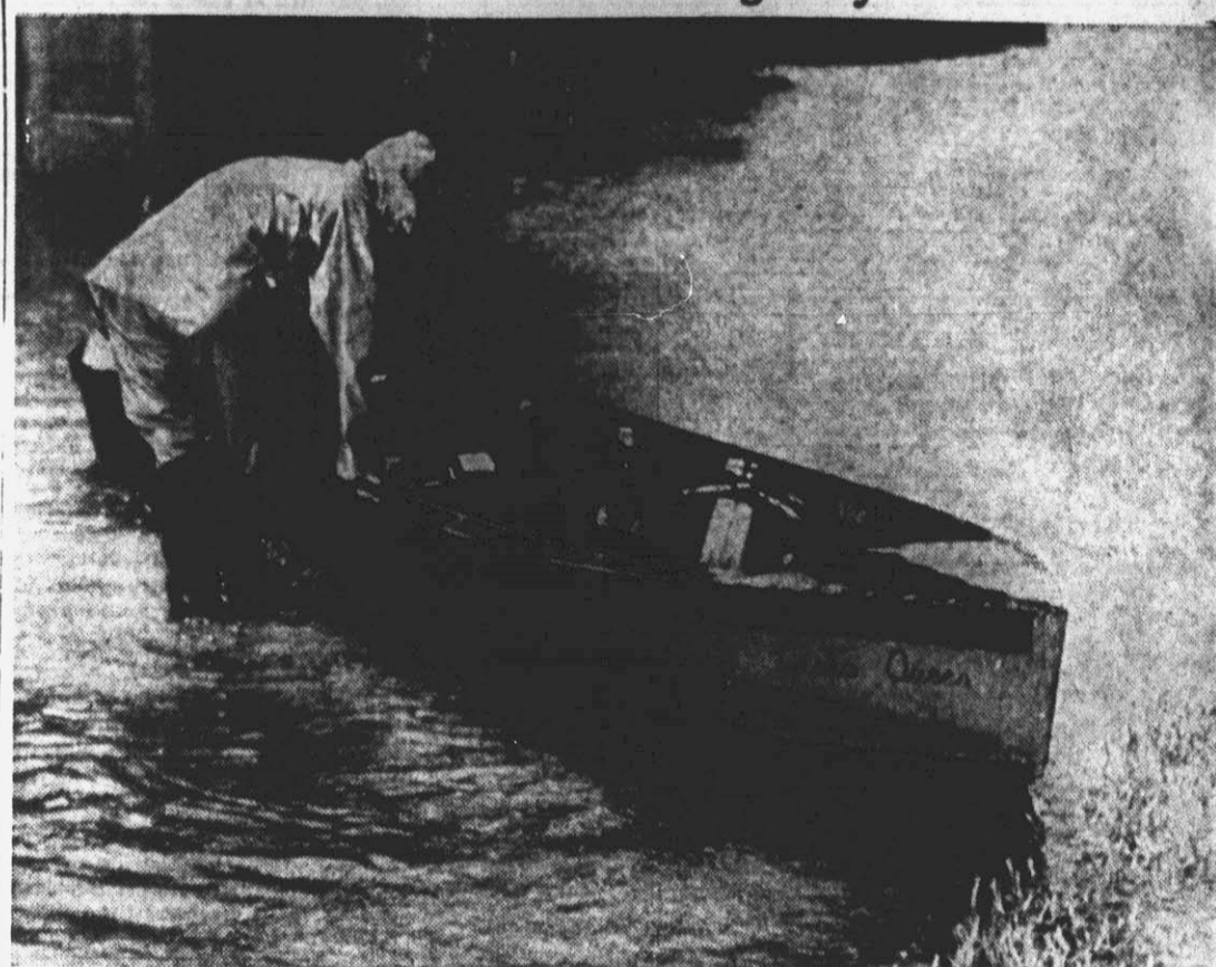
FERRY SERVICE?—Getting back and forth to Wilson's Store on the New Bern highway was accomplished only by boat yesterday afternoon. Waters from flooding Green Mill Run blocked the highway and surrounded the nearby store. Above Johnny Wilson, operator of the business, is shown as he casts off from the north "bank" of the stream to make the trip to his establishment. (Reflector Photo by Alvin Taylor).
