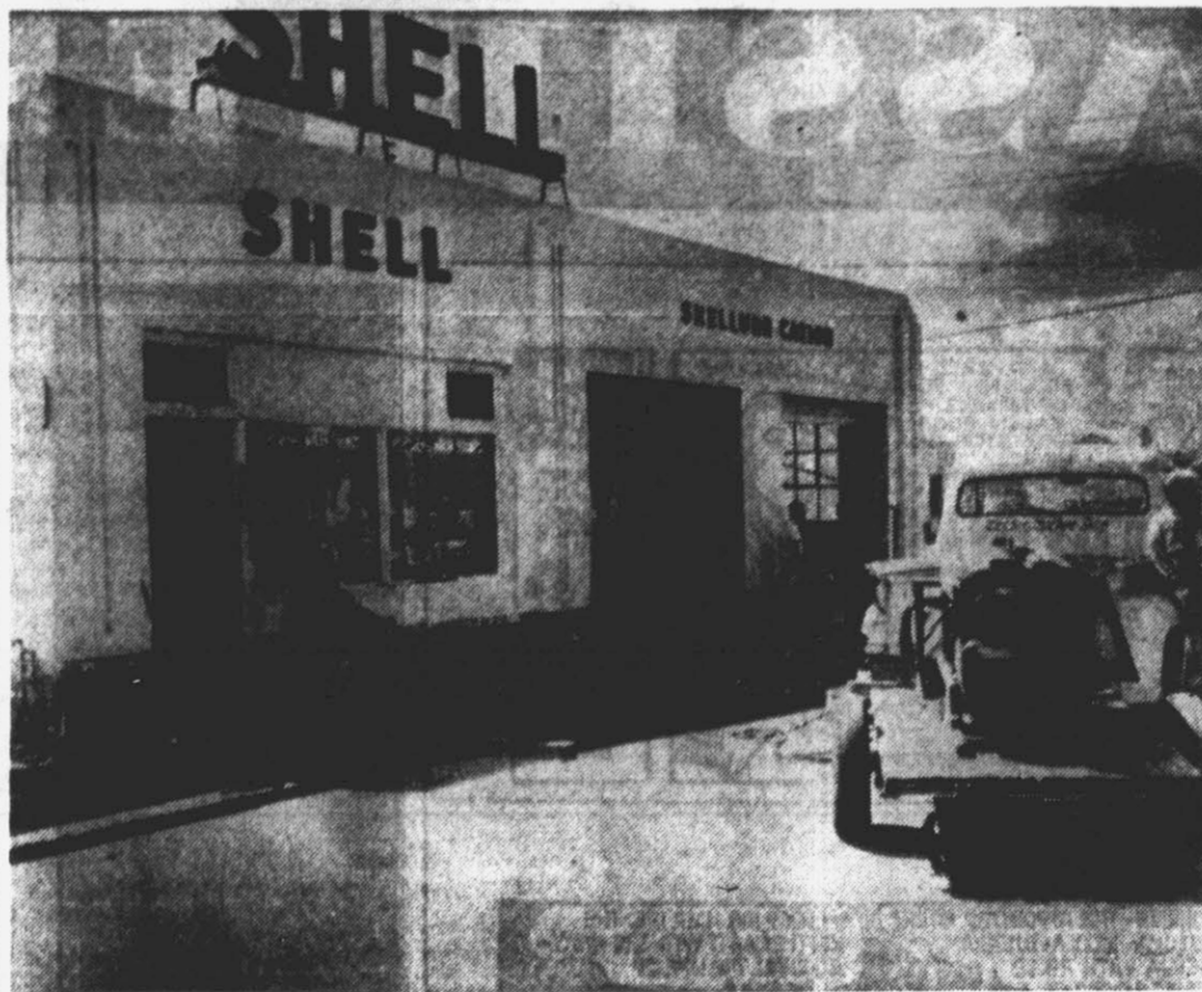
This service station at West End Circle is being moved back from its present location to make room for the new traffic circle which is to be constructed at that point to channel traffic from the three highways which will intersect there when the new N. C. 11 bypass is completed. A number of other buildings at the intersection must be moved to make way for the improvements. (Reflecto Photo by Alvin Taylor.)
