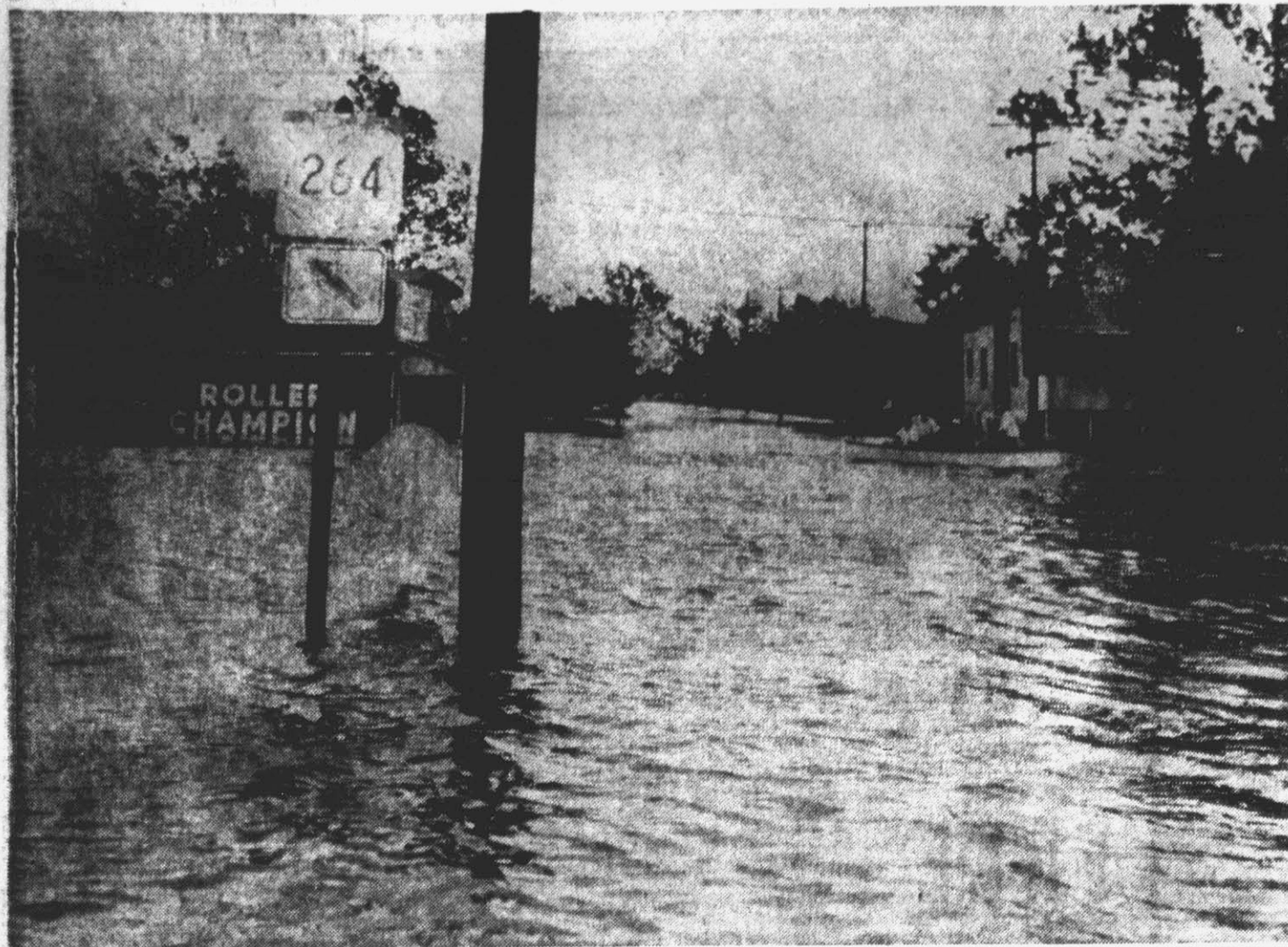
FLOODED INTERSECTION—A boatload of people (extreme right) move into an intersection at US 264 east in Washington yesterday while in the foreground a directional sign and a stop sign rear above water. In the background, water laps against the side of a store. Depth of the water at this spot reached six feet in places. (Reflector Photos by Bob Hilldrup.)
