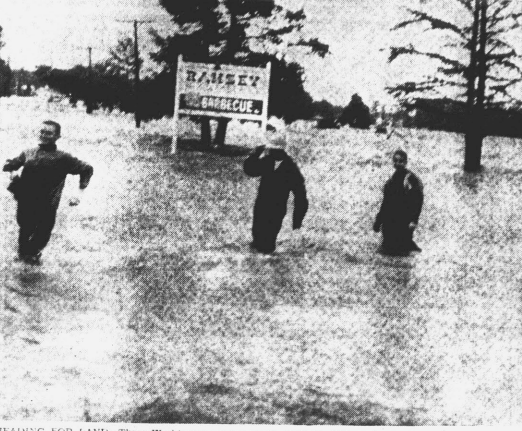
HEADING FOR LAND—Three Washington youths battle through high water to land after inspecting damage at a barbecue stand near the National Guard army. Behind the youths a highway bridge and a railroad trestle are covered with water.
