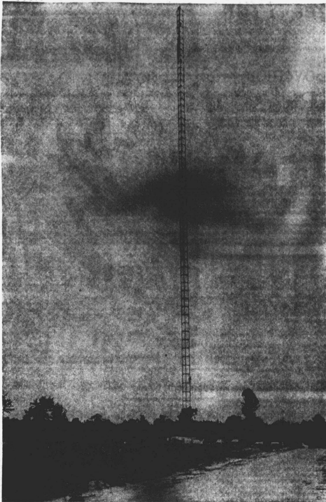
Now going up on the outskirts of Grifton is a transmitter for WITN television, located in Washington. When completed the tower will stretch 921 feet above ground. The Washington tv station will be operating on 316,000 watts. It has been assigned Channel 7 and will be affiliated with the NBC television network. (Reflector Photo by Edwina Haymes.)
