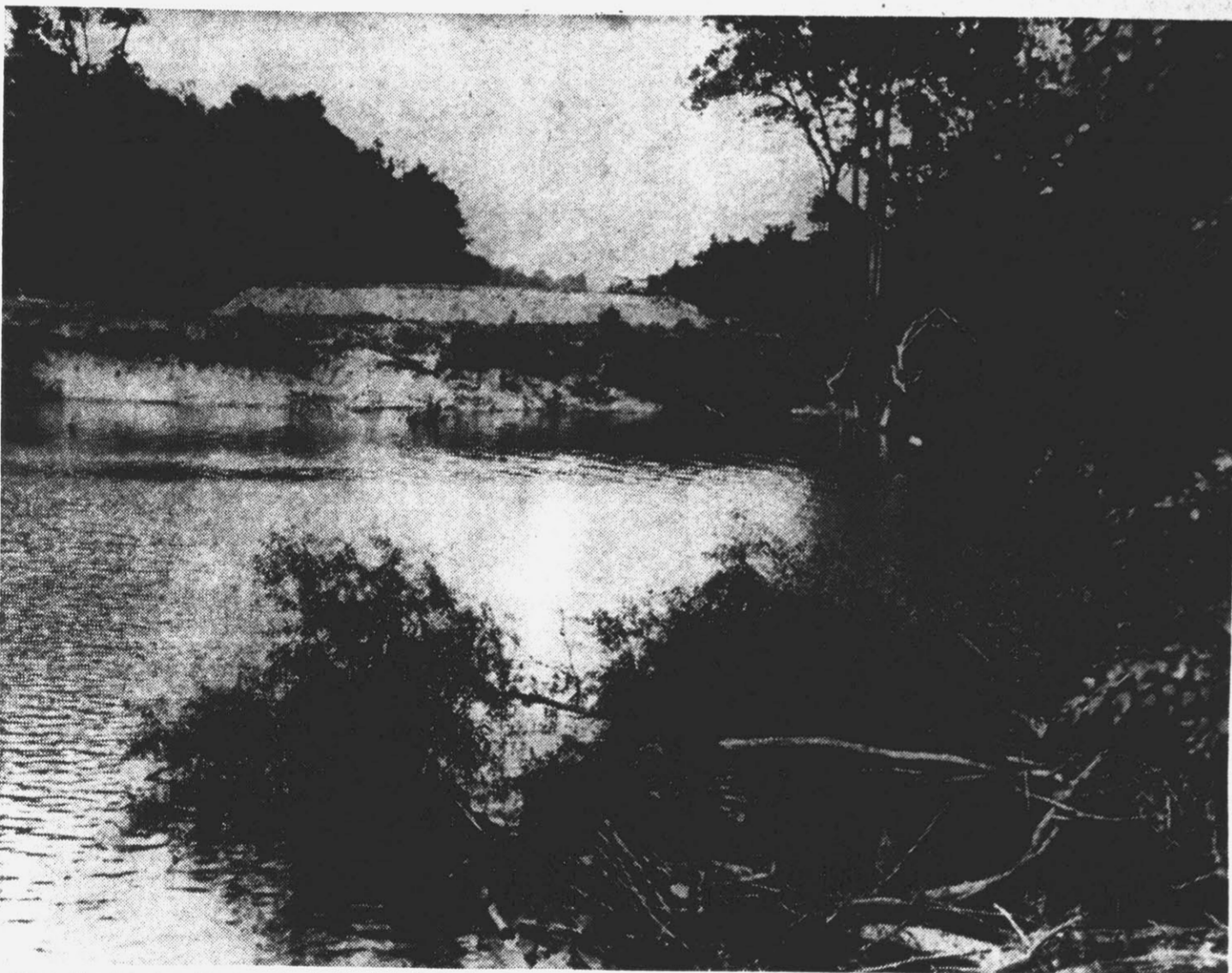
This is the site where the new river bridge is to be built. On the far bank of the river can be seen the fill which will lead to the bridge. From this point the highway will cut across low land to intersect with the present Memorial Drive. (Reflector Photos by Alvin Taylor.)
