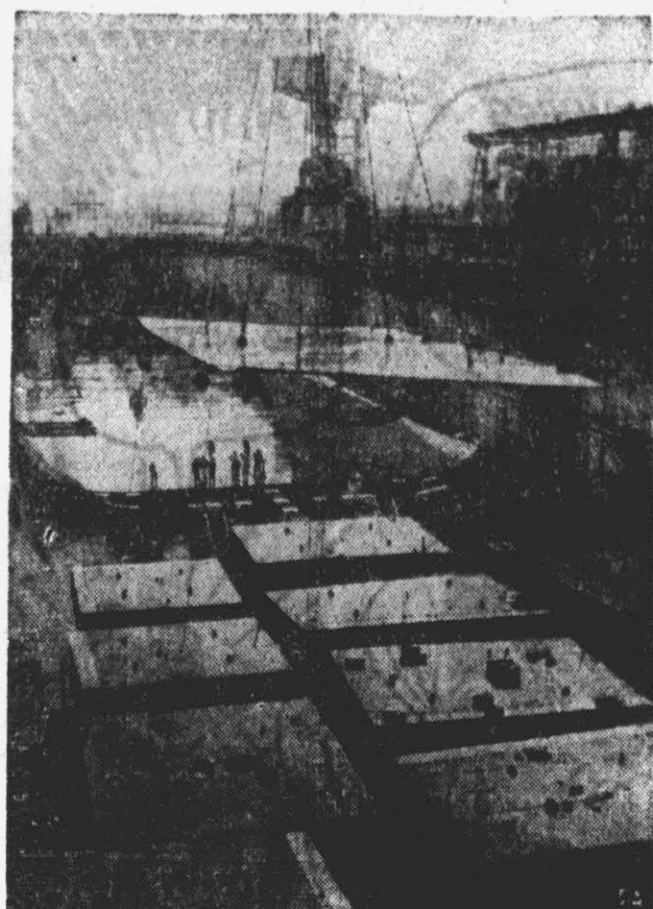
CARRIER A-BUILDING — Keel plate for new Forrestal-class 60,000-ton, 1,046-foot long aircraft carrier independence is laid down at N. Y. Naval Shipyard, Brooklyn.
