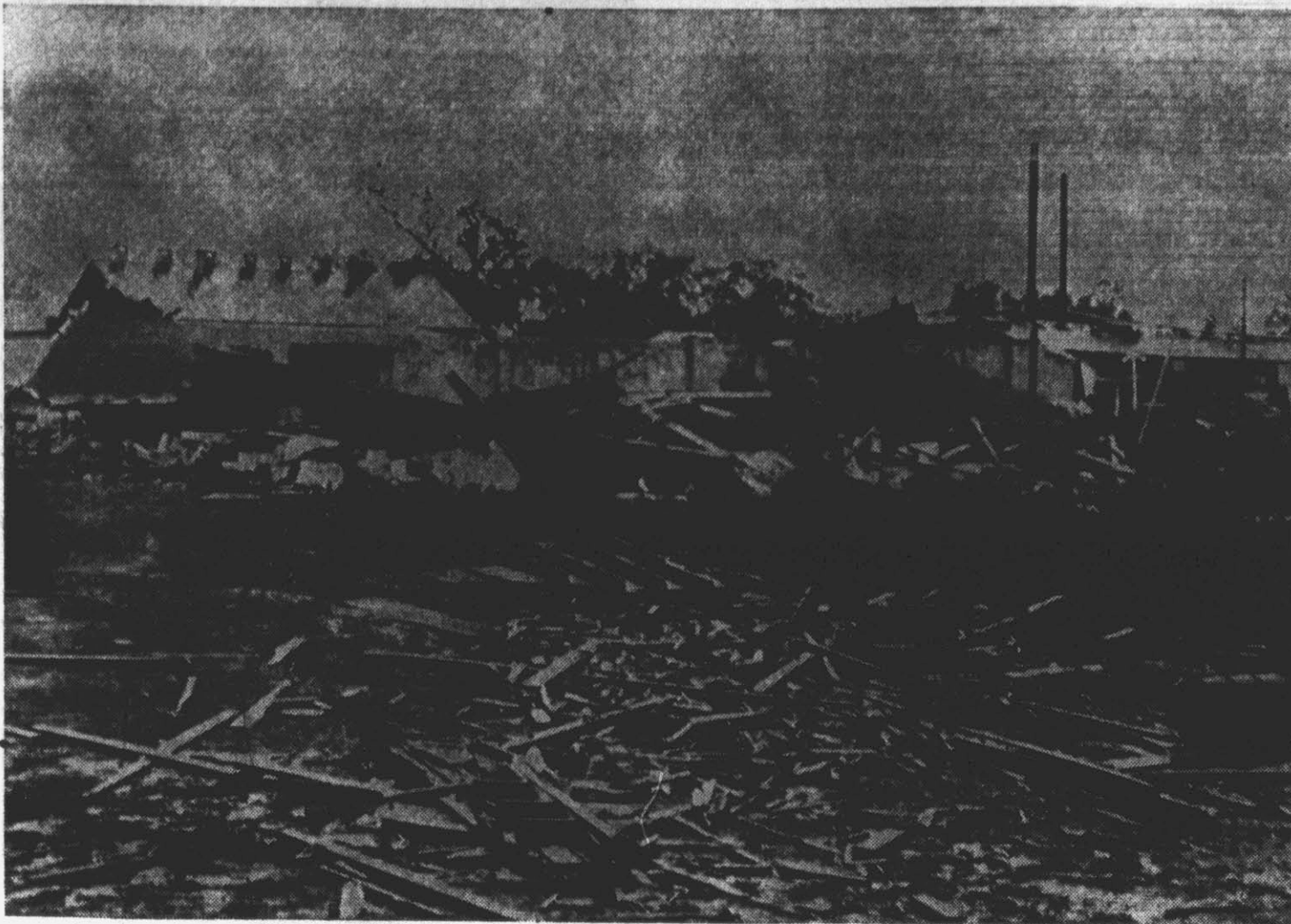
When Saturday's tornado struck this potato house on the eastern side of Bethel it completely leveled the building and scattered debris over a wide area. Located directly behind this building is the Bethel Auction Market which partially collapsed when a concrete wall was blown down. (See other picture, page 12.)
