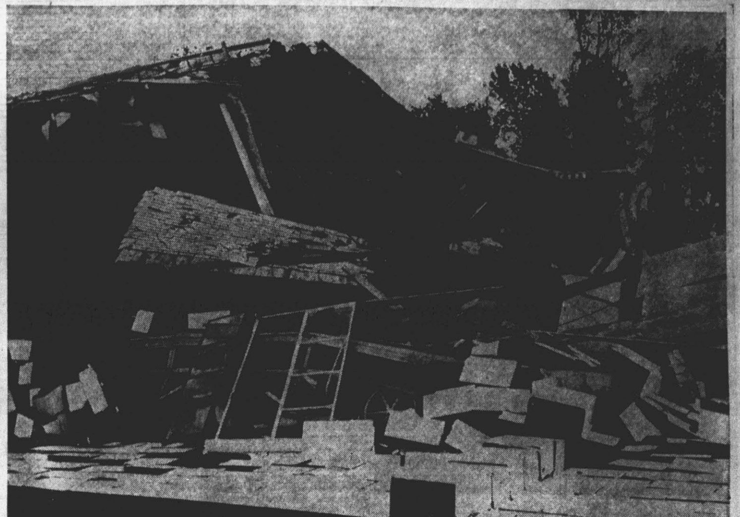
The above pictured potato house, one of two belonging to J. R. Cullifer, was completed only last October. The building was leveled by Saturday's high wind except for the small section shown in the background. Potato grading machinery in the building was believed to have been heavily damaged. (Reflector Photos by Alvin Taylor.)
