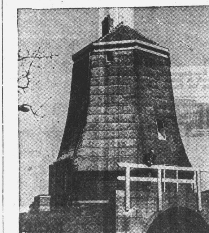
LOWLAND CONVERSION — This house, a former windmill near Utrecht, shows Dutch ingenuity. Sails were removed, sides were thatched with chimney and windows added.
