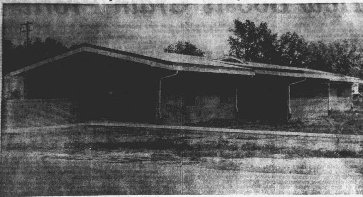
NEW AYDEN CLINIC OPENS—A new, $40,000 medical clinic will open Monday in Ayden, headed by Doctors L. M. Alexander and Clifton Davenport. The new building will include a reception room, offices for physicians, examining rooms, an x-ray room and utility rooms. (Reflector Photo by Alvin Taylor.)
