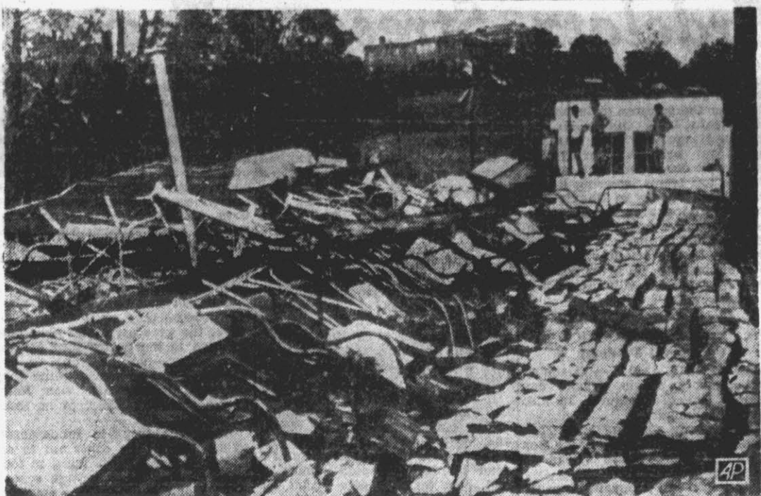
TORNADO STRIKES CHILDREN'S HOME —Youngsters living at the Masonic Children's Home survey their demolished milking barn which was struck by a tornado at Macon, Ga. About 200 children escaped injury as the storm unroofed a dormitory of the main building shown in background. No deaths have been reported but damage in the area is estimated at a million dollars. (AP Photo)
