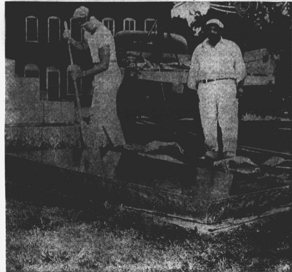
Workers are shown above as they put the finishing touches on a memorial to World War I and II and Korean War dead from Pitt County. The stone is to be dedicated in ceremonies beginning at 11:15 a. m. next Monday. (Reflector Photo by Alvin Taylor.)
