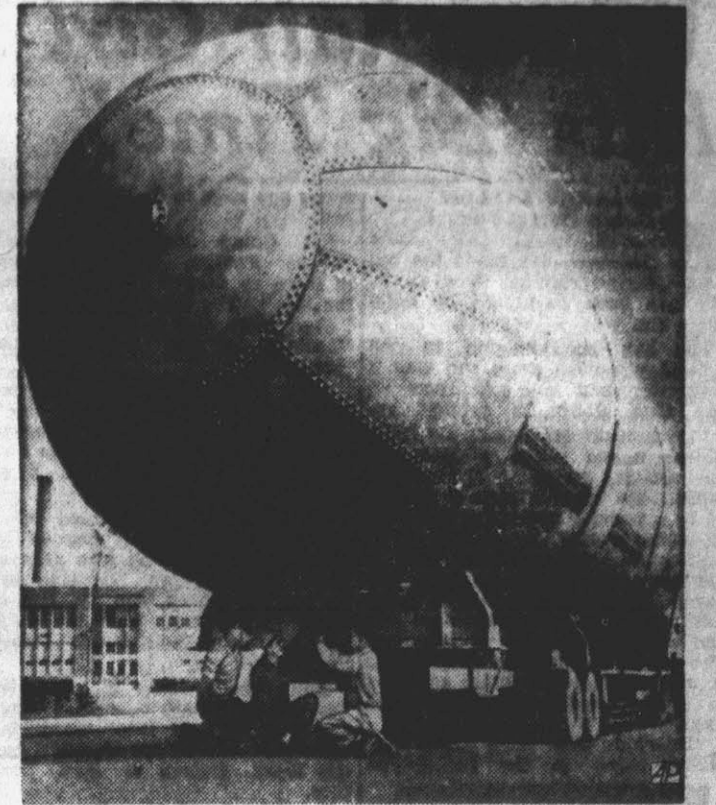
HEDGE-HOPPING BLIMP?—Despite appearances, this is no low-flying blimp, but a 30-ton, 57-foot-long, 17-foot-high gas storage tank being moved through Philadelphia.
