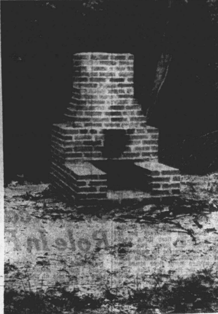
Four outdoor fireplaces have been constructed at the park, and picnic tables will soon be set up there. (Reflector Photos by Edwina Haymes.)
