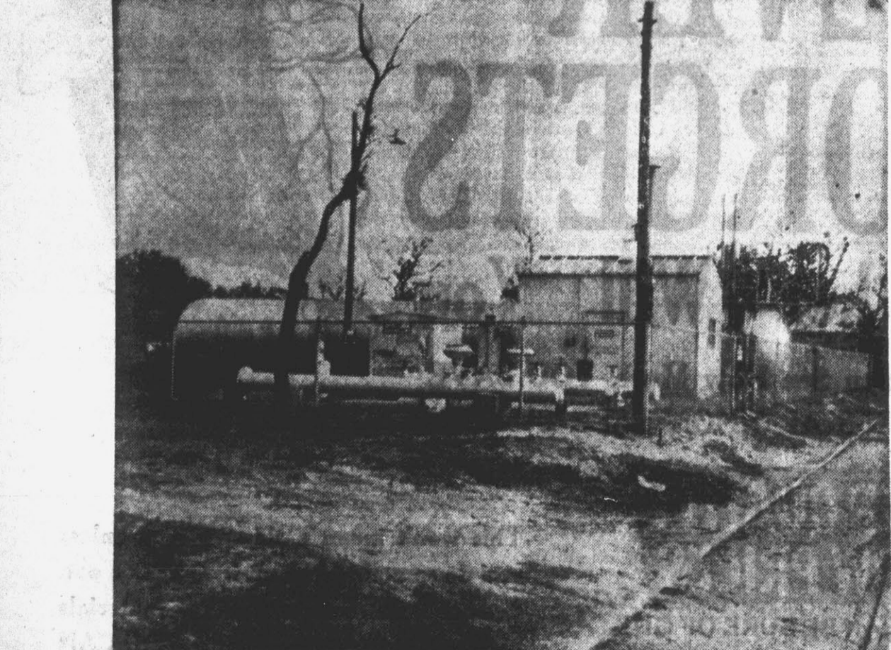
Thirty Years of Service WITHOUT UPKEEP. This Stewart Fence was Erected in Greenville Over 30 Years Ago and Is Still in Use on this Property of the Greenville Utilities Commission. A Close Inspection Shows No Rust Spots, No Deterioration. It's Still As Good As New.
