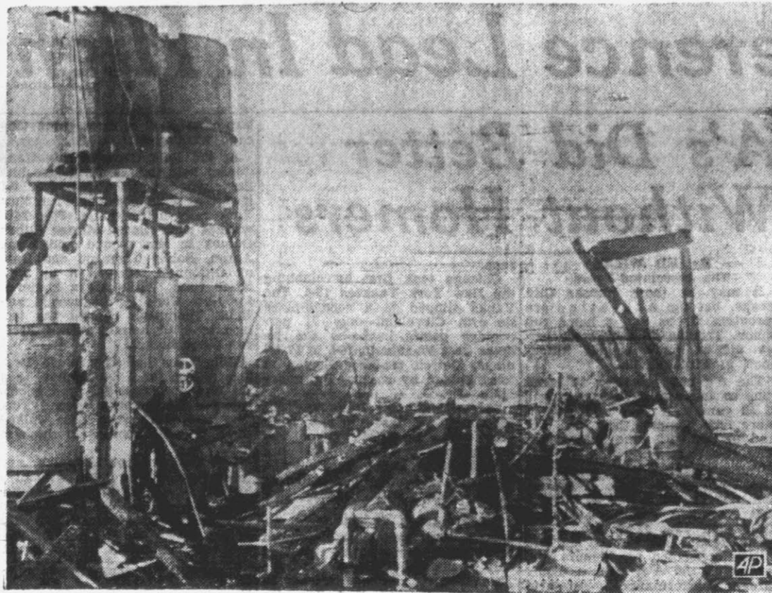
BLAST WRECKS CHEMICAL PLANT. —Several tanks, pipelines and charred timbers remain after a series of blasts wrecked the Crescent Chemical Co plant at New Orleans. The explosions rocked the downtown area, damaged several houses and set fire to the Galvez Street wharf. Damage to warehouse and contents was estimated at $50,000 while the wharf fire destroyed some $7,000 worth of pilings. (AP Wirephoto).
