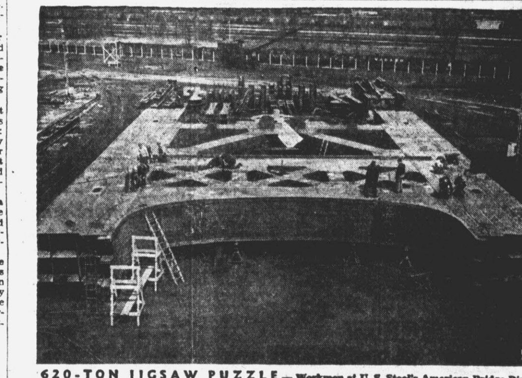
620-TON JIGSAW PUZZLE —Workers at U. S. Steel's American Bridge Division, Gary, Ind., put together and "match mark" a section for Mackinac Bridge in upper Michigan.
