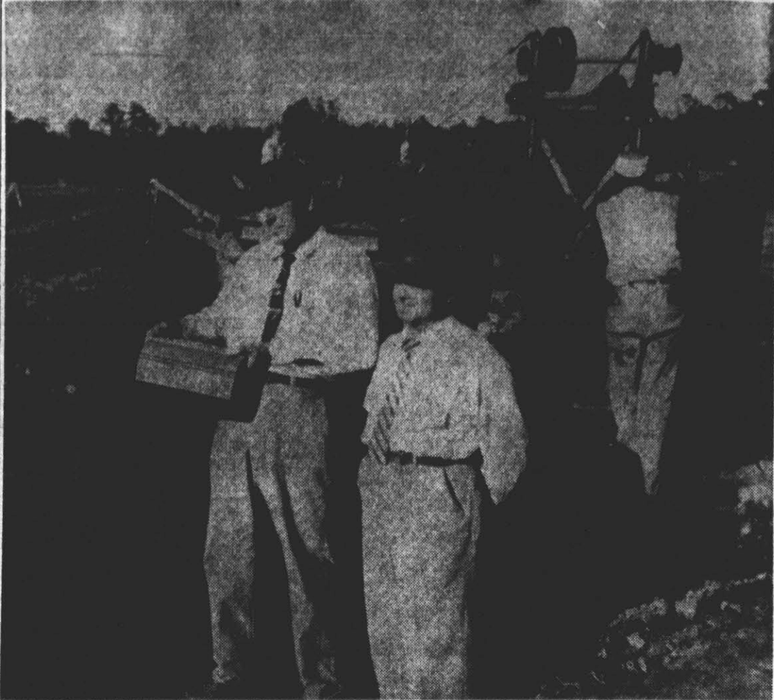
Julius Parker, who supervises the work of two drainage tile laying machines, is shown above as he holds the two millionth tile to be laid in Pitt County. Looking on is Jack Lewis on whose farm the tile was laid. (Reflector Photo by Alvin Taylor).
