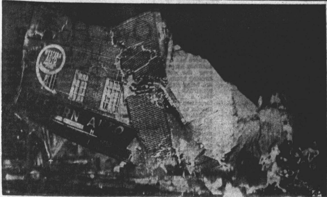
DEATH OF A BUILDING:—This brick store, ravaged by a fire that swept Bowling Green, Va., comes down with a roar as the fire burns on. Twenty-five business buildings in this little community of 700 persons, were destroyed or badly damaged by the fire. High winds, fanning a brush fire, swept the blaze into a barn on the edge of the business district to start the wholesale destruction. (AP Wirephoto).
