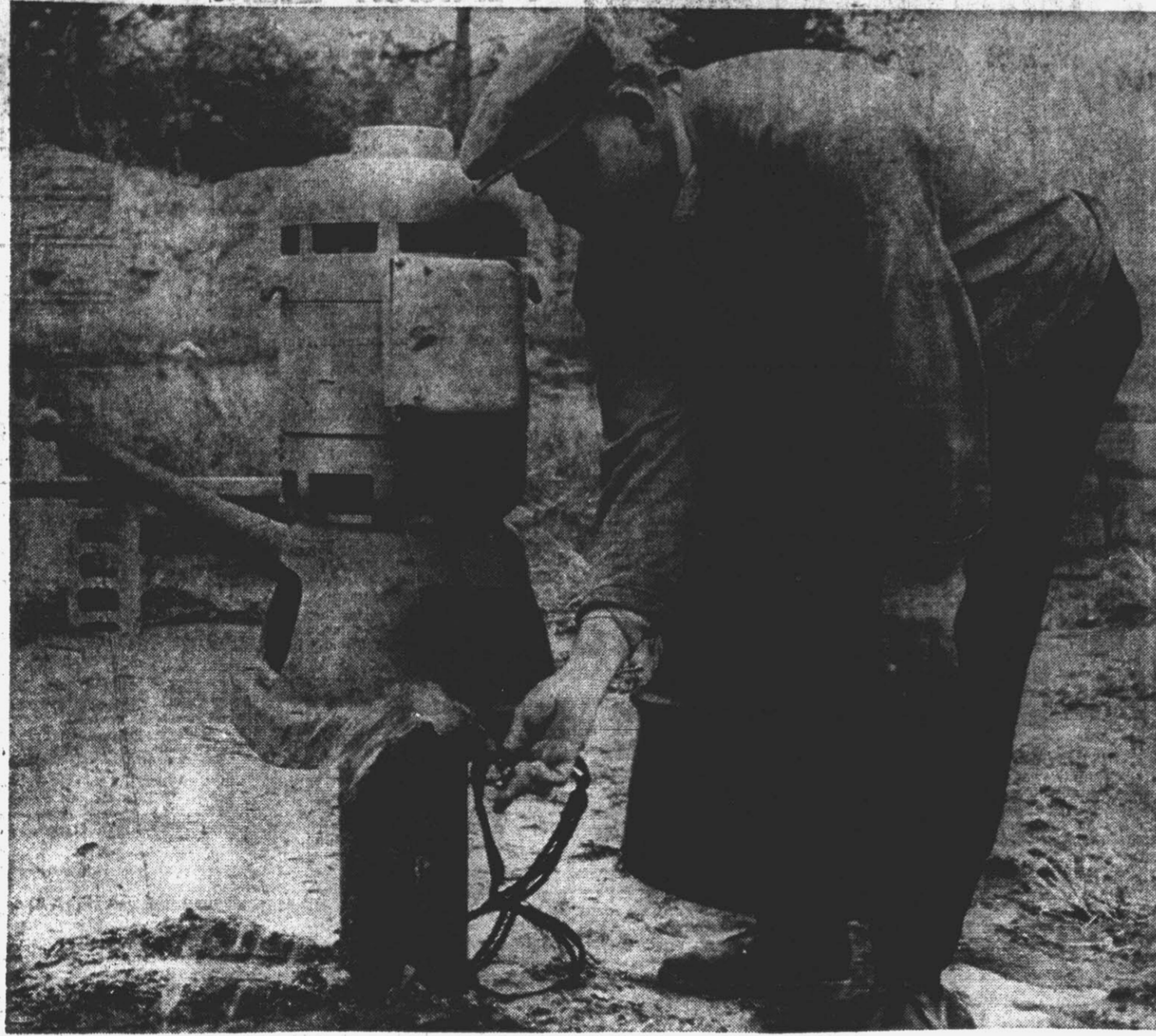
DEEP WATER: — Don Langston of Winterville gets a drink from his irrigation well. The gravel-wall well goes down 407 feet and can supply water at the rate of 450 gallons a minute. The well-water is pumped into a large reservoir which furnishes water to two smaller ponds, from these Langston can irrigate 40 acres. This type of system is recommended in eastern North Carolina. The state's first 1955 irrigation demonstration, conducted by the State College Extension Service, was held on the Langston farm Tuesday. A total of 27 demonstrations will be held in the state this year. (Photos by Ralph Mills).
