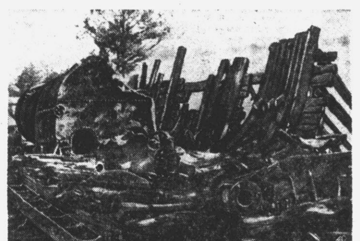
OUT OF THE MUD — view from the stern of the C.S.S. Pee Dee showing the dual fire boxes of the boiler and the network of beams in the hull.
